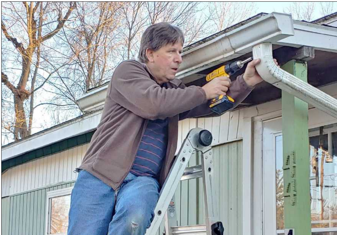
A LifePath Home Repair Program volunteer fixes a rain gutter.
